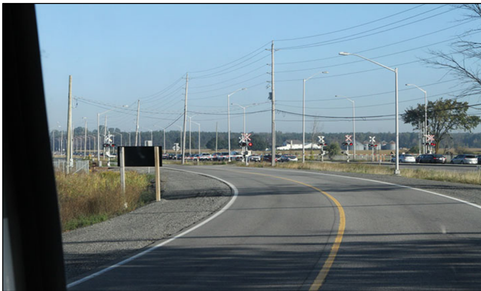
Photo 11. Crossing lights on Woodroffe Avenue and on the Transitway were fully visible when the bus was 402 feet (122.5 m) from the Transitway crossing (see location 4 on Figure 7)
