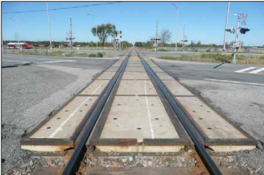
Photo 7. Looking eastward from the west end of the crossing, train wheel flange marks were observed from the middle of the crossing extending westward
