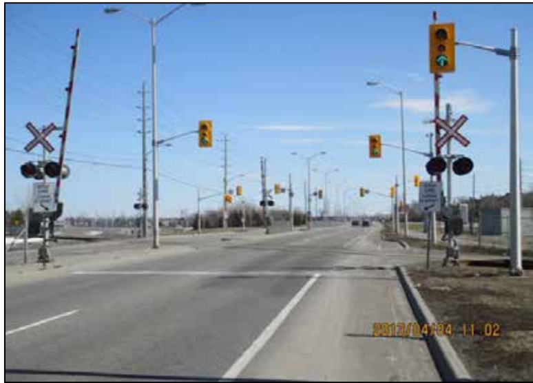
Photo 15. Fallowfield Road looking east (Source: Jock Valley Engineering)
